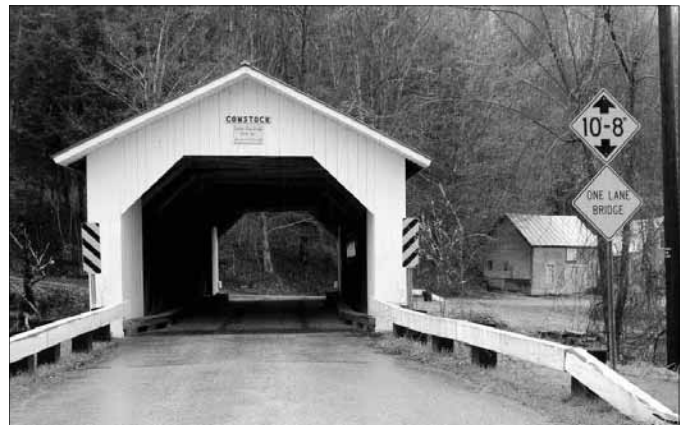
Figure 13. Comstock Bridge, Montgomery, VT. Photo by Ken Secor
