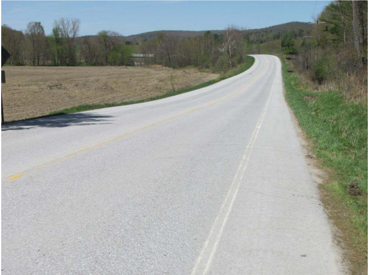
Figure 14. RT 118 looking north toward Longley Bridge (on left behind trees). Note riparian buffer on upper left (photo: Bob Hawk, 5/7/12).
