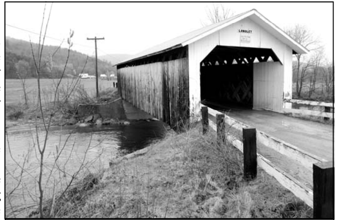
Longley Bridge—Trout River
