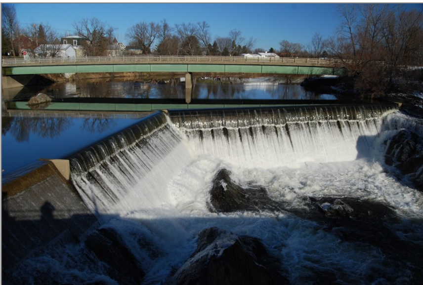
40. The dam and falls at Enosburg Falls, taken from the historic Bridge of Flowers and Light (photo by Shana Stewart Deeds).
