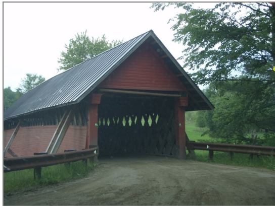
16. River Road covered bridge, off of River Rd. in Troy (photo by Shana Stewart Deeds).
